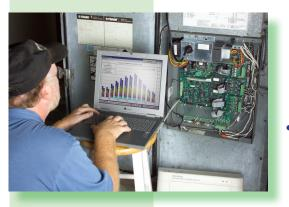
(electricity, natural gas, chilled water, etc.). At the simplest level, one can record total building energy use on a daily basis. At a higher level, energy use can be recorded in time-of-day format. For further analysis effectiveness, consider submetering specific energy end uses such as HVAC equipment, reheat, lighting systems, or others, which can help to disaggregate failures or dysfunction for specific equipment or subgroups of equipment.
